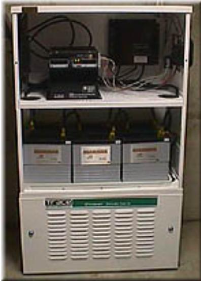
**Inverter & 12 Batteries** After the first great ice storm, we added a separate inverter/battery system as backup for the times the grid power is down. Since our main intertie inverter system depends on grid power to work, we have a second system to handle those few but critical times when the power is out.
